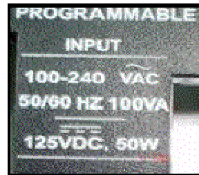
Fig 2 : The incorrect marking of front plate
